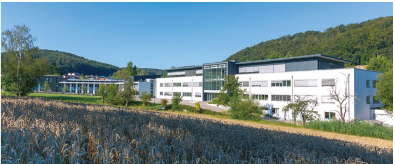
The company headquarters of REA Elektronik GmbH, 30 kilometers south of Frankfurt am Main, Germany
