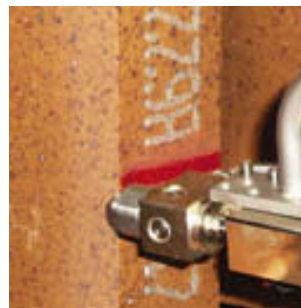
Chimney stone line-marking for correct installation
